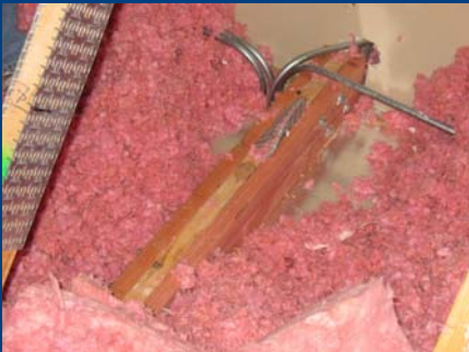
Install New Bolted Repair
