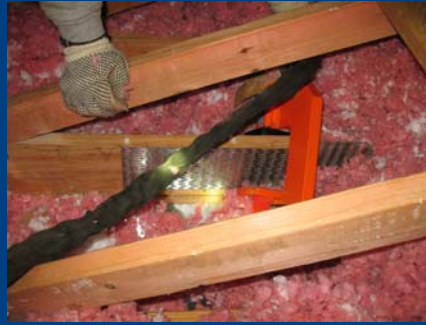
Install New Connector Plate
