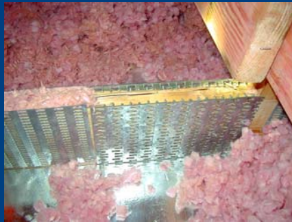
Install New Connector Plate
