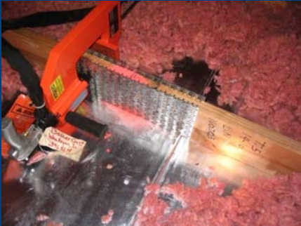
Repair: Install New Connector Plate
